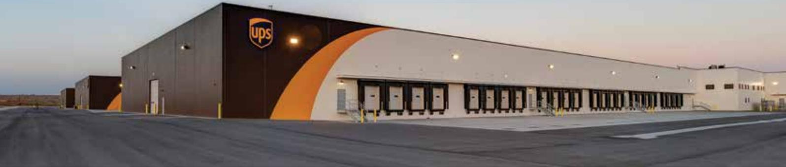
The perimeter of the main building is more than 1.3 miles long with 25-ft. high tilt-up concrete panels. Crews placed an average of 40 panels a day during peak construction activity. The project is located in the heart of the proposed 'Inland Port', one of the more hotly debated future projects in the state currently in its infancy. (photos courtesy Layton Construction)
